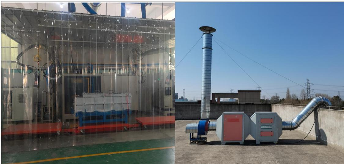
软帘封闭发泡区+集气罩+两级活性炭吸附装置+15m 高排气筒
